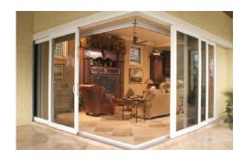
**Pocket Doors:** This feature allows the sliding glass panels to retract into the wall or merely hide out of site behind the wall. The benefit is that you have an opening completely void of everything but the view.
